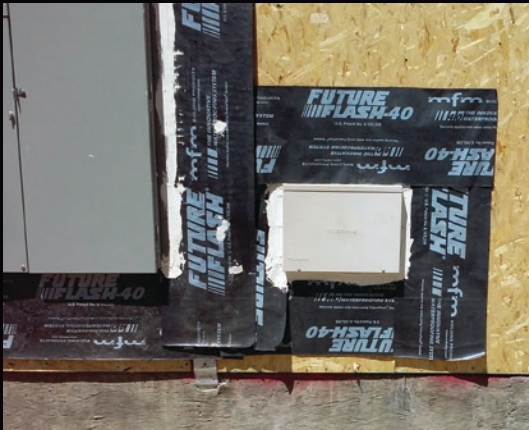
FutureFlash® offers high strength, high elongation and is flexible to accommodate expansion and contraction of the substrate.
